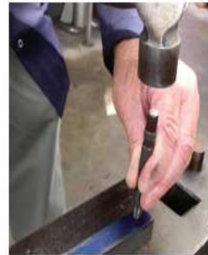
Use a rule to re-check the marked position. Center punch the location of each hole ready for drilling.
